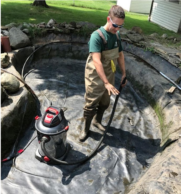
Removed all vegetation, vacuumed clean
